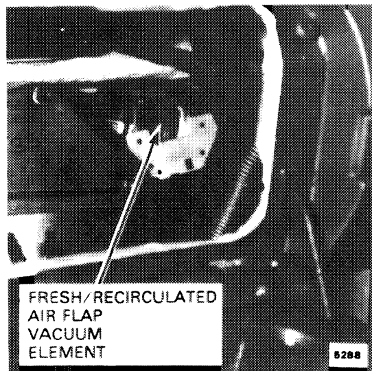
Figure 4 - Behind Glove Box
